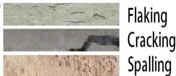
Fig -29: Flaking, Cracking, And Spalling
