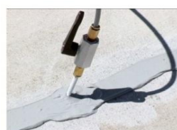
Fig -11: Crack Repair by Gravity Filling
