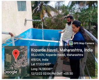
**3. Filtration Media**: In this stage water comes in the filtration beds through tube settler. In this stage water can passes by filter bed consist of sand gravels of various sizes
