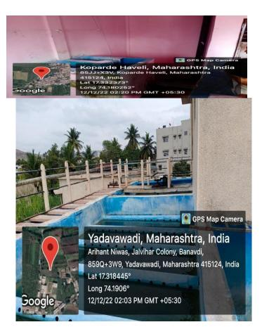
5.Storage Tank: After disinfection of water pure water collects at underground storage tank.
