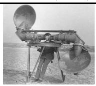
Before the air defense came out, a specially trained person warned that enemy aviation was coming. He worked with a special "gadget". Large acoustic windows focused on the sound, amplified it, and helped to hear the sound of the engine.
