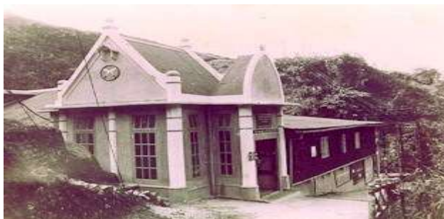
Figure 4: Sidrapong Hydel Power Station
