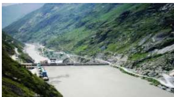
Figure 7: Nathpa Jhakri Dam
