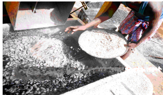
Pic no.05: Shredded plastic waste is added
