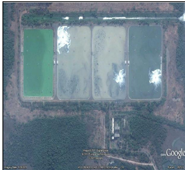
Figure 13: Location of Ghatkopar Lagoon Works Embankment
