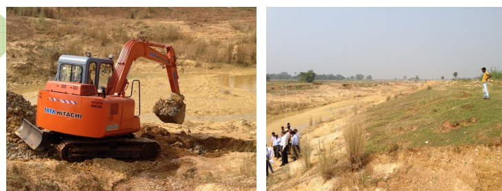
Figure 3 Investigation team at the Problematic Reach
