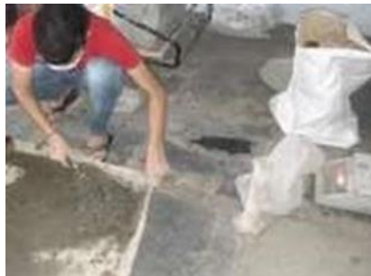
Fig. 5. Mixing of concrete
