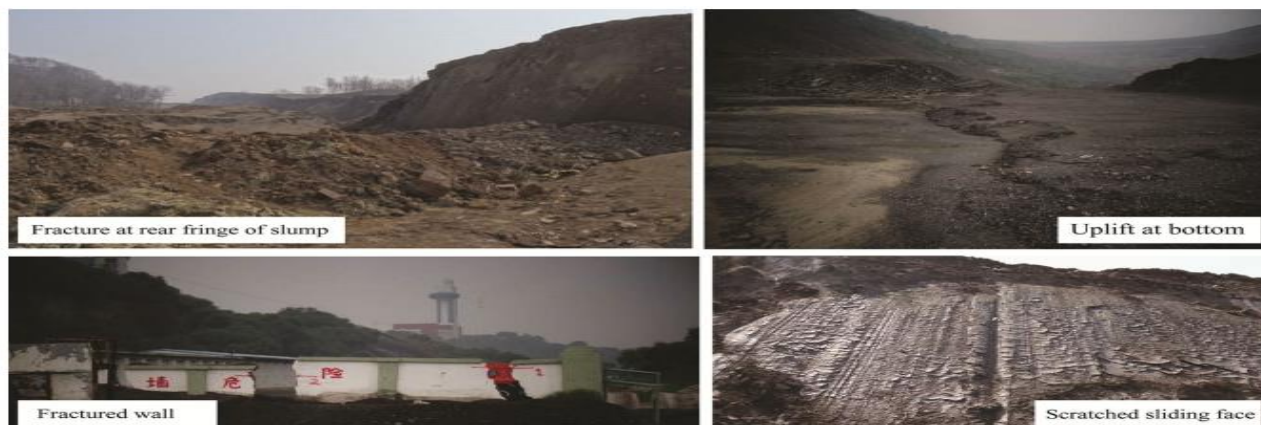
Fig. 4 Landslide-induced surface phenomena
