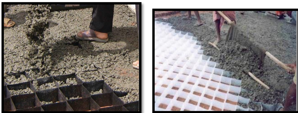
Figure.3.- Application of plastic cells during road construction
