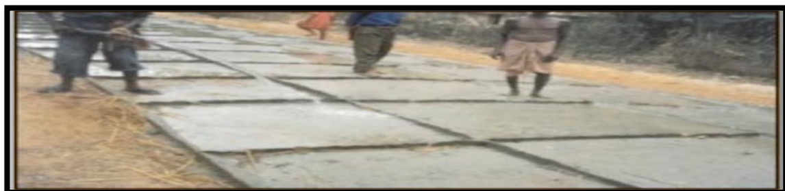
Figure.4 Wet paddy straw and ponding used to cure concrete
