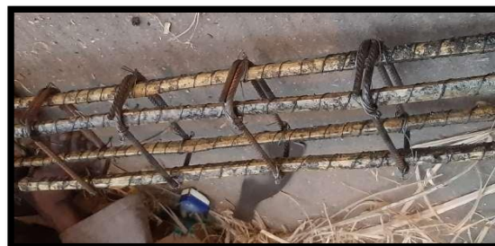
Fig. 3. Treated Bamboo reinforcement
