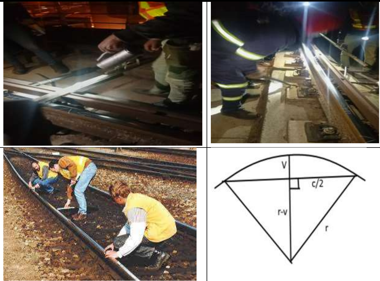
Figure 4.2-1 Illustrations of Gauge adjustment tools and principle
