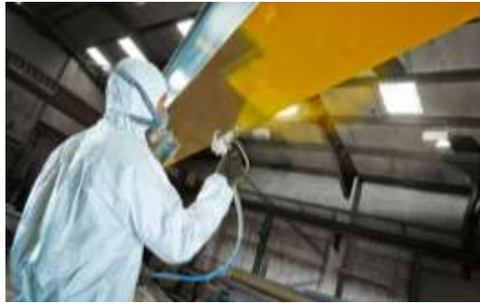
Figure 5. The spray gun coating
