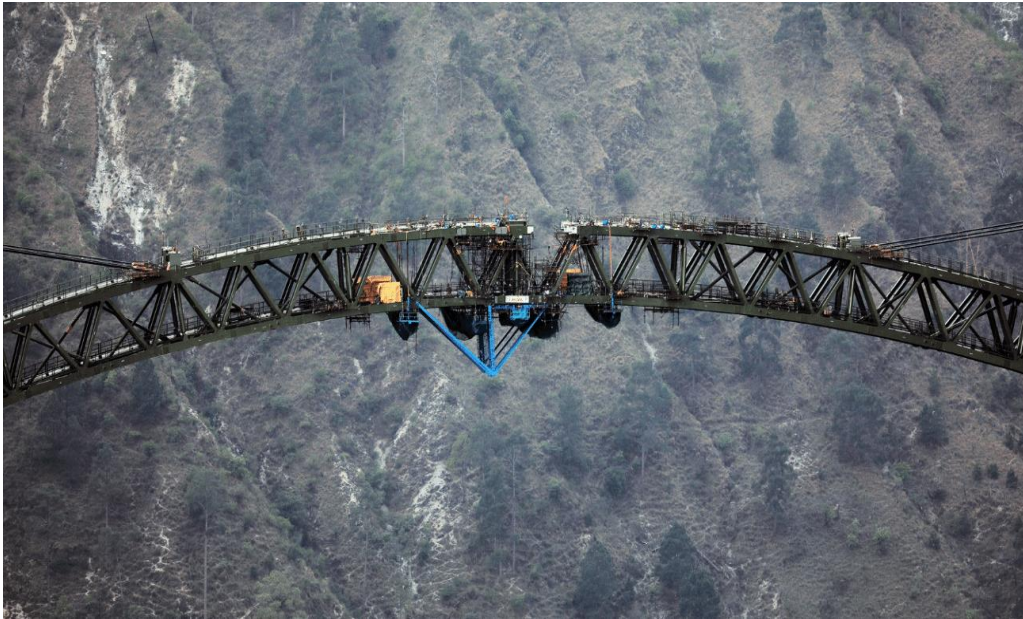
Figure 6: Connecting the both levels of arch
