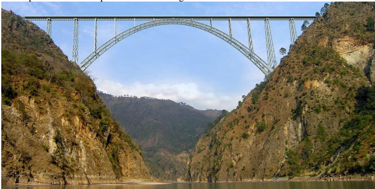
Figure 1: The Chenab bridge when completed
