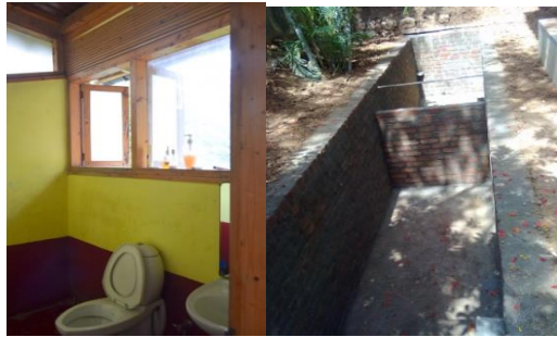
Fig. 4. Reused sanitary fittings Fig. 5. Rain water sump
