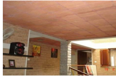
Fig. 12. Hourdi blocks as heat insulator
