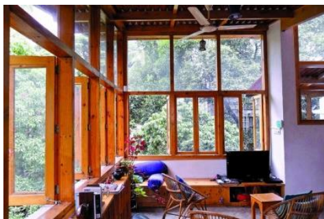
Fig. 7. Large reused windows
