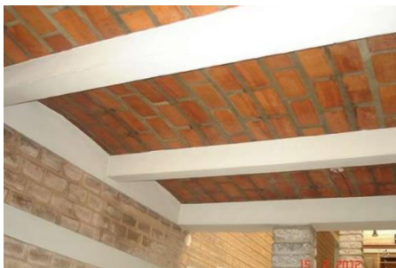
Fig. 11. In-situ Jack arch roofing panels
