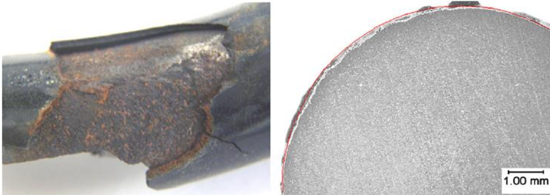
Fig 5 Coil spring which broke due to corrosion[1]
