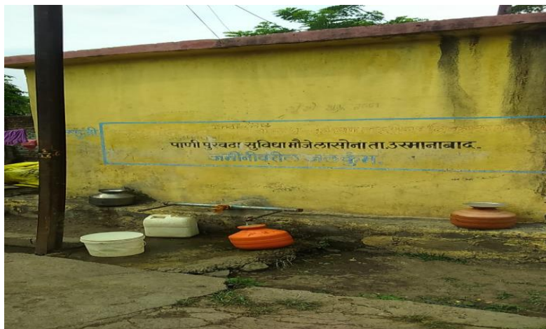
Fig 1:- Present water supply arrangement
