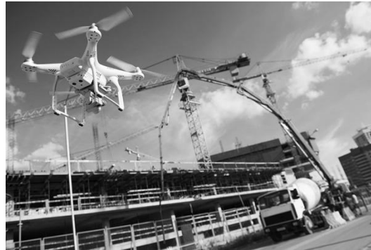
Fig.2: Use of drone for construction sites
