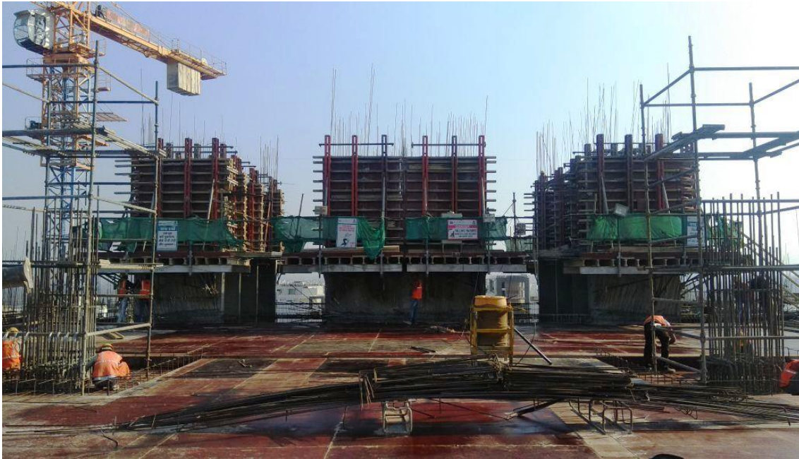
Figure 9: Elevation of Jump Formwork system on site
