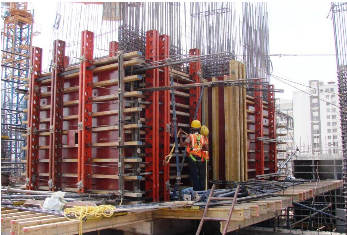
Figure 10: Fixing of Superslim Soldier in Jump Formwork system on site
