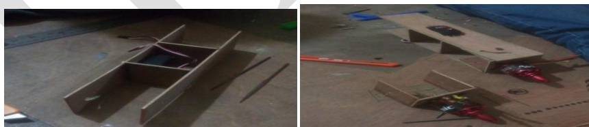
(Figure 7.4: Construction of tilting frame and motor mount)
